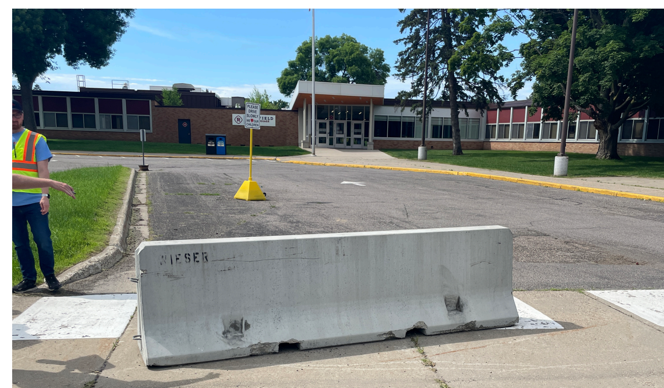
Barrier to manage access at school entrance Barrera para controlar el acceso a la escuela
