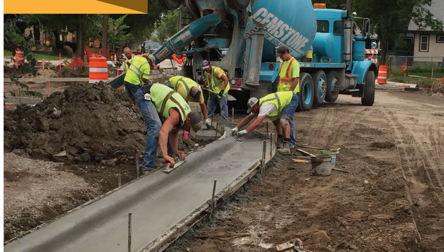
5 CURB + GUTTER INSTALLATION
