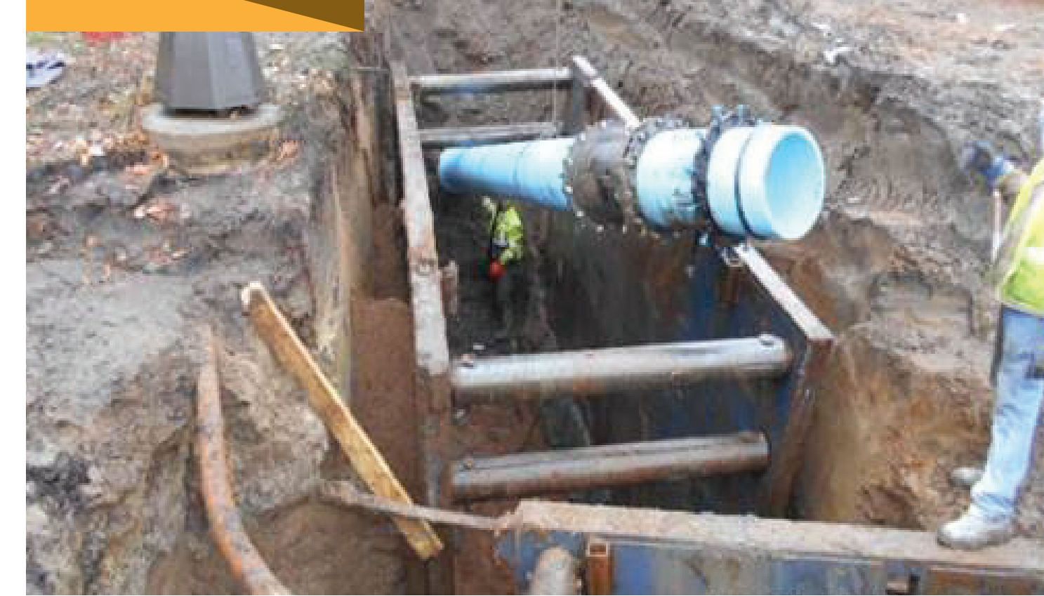
3 WATER MAIN REPLACEMENT
