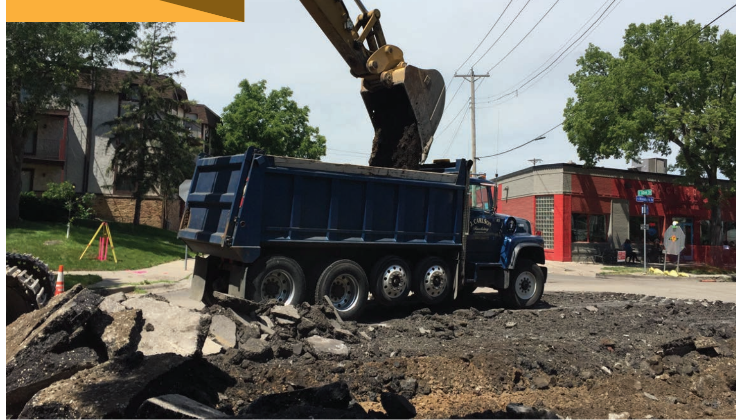
1 PAVEMENT REMOVAL
