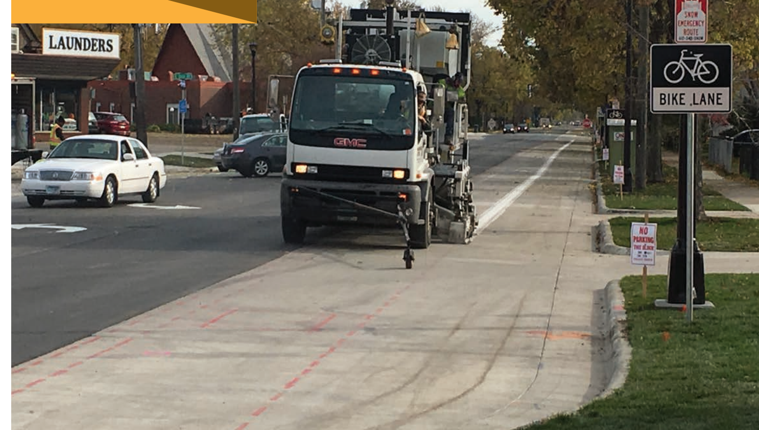
6 ASPHALT PAVING + STRIPING
