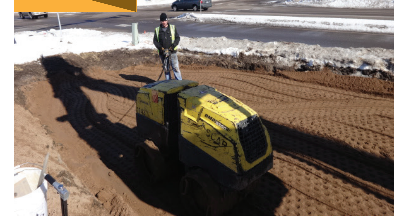
4 SOIL REPLACEMENT + COMPACTION
