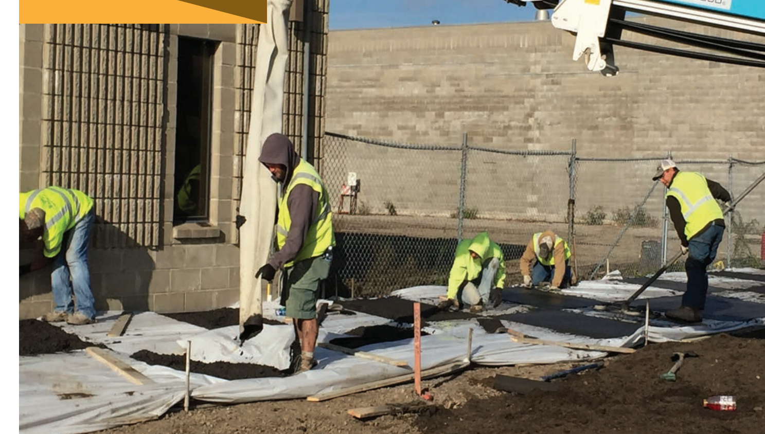
7 SIDEWALK + TRAIL REPLACEMENT
