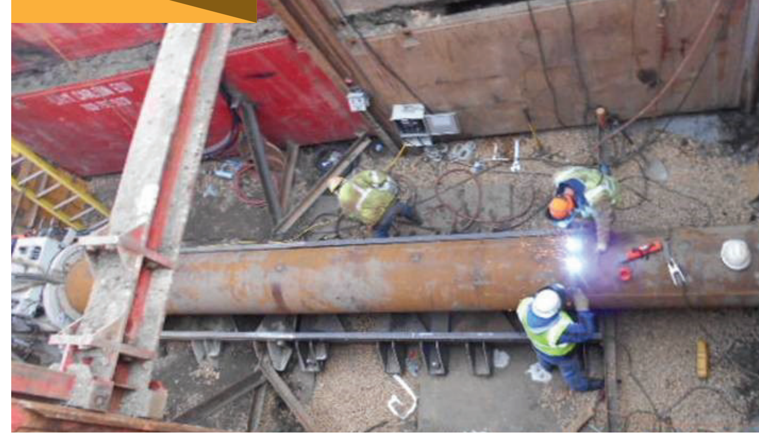
2 STORM + SANITARY SEWER REPLACEMENT
