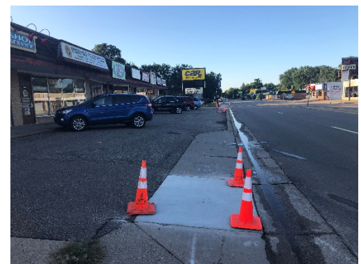
Missing sidewalk along Penn Avenue
